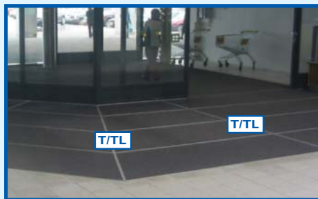
Frames of different widths used as dividers for large left to right installations of 9/16" matting.
